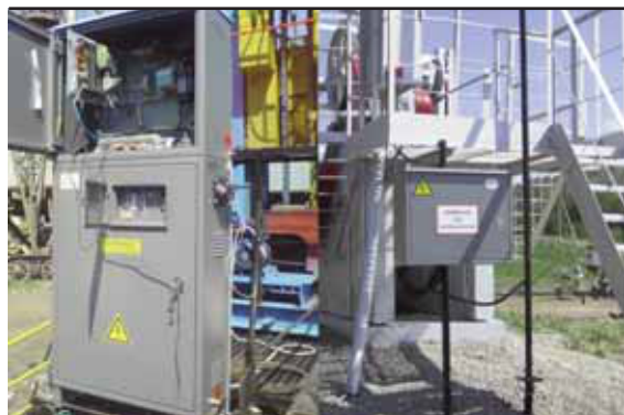
Fig. 4. WellSim controller with Power control station
