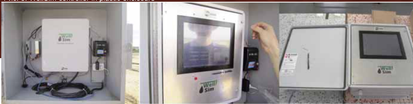
Рис. 5. WellSim controller in plastic enclosure
